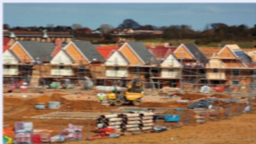
▲ Construction at a building site
